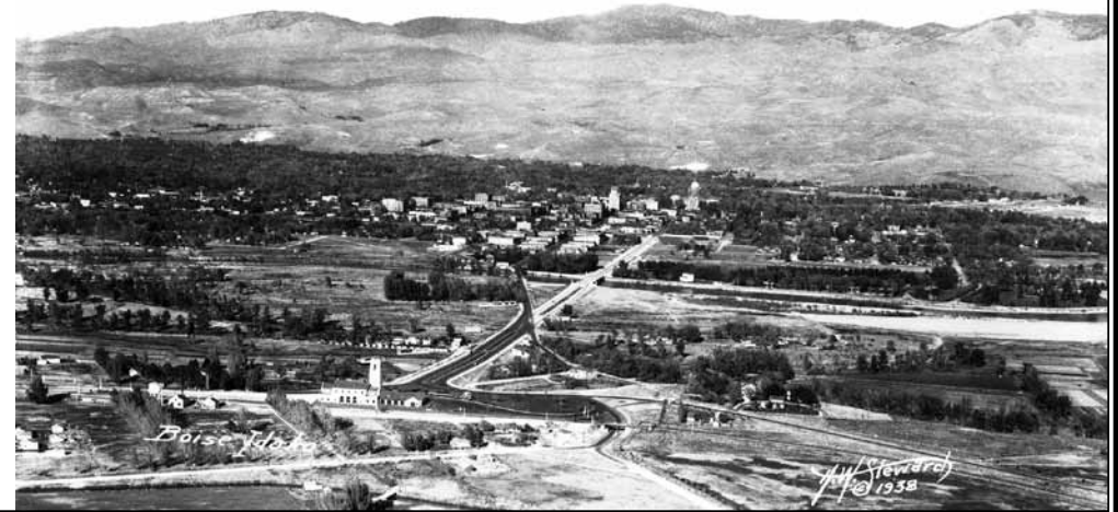
1938 aerial view of the Bench looking north—note Hulbe Drive to the right of the depot (Idaho State Historical Society, 72-190-35a).
