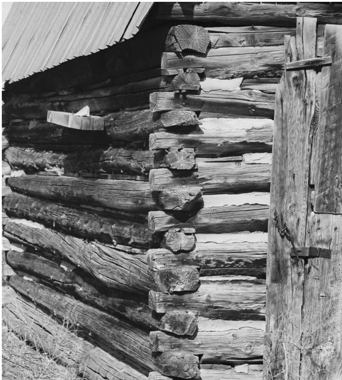
Above: The barns exhibit corner notching that appears to be a cross between square and double notching.
