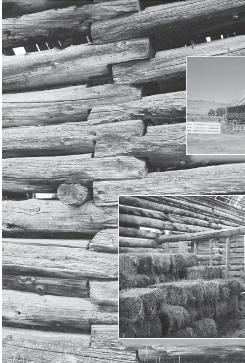
Large photo: A view of the spliced logs on the south side of the barn. Bottom right: The log partition inside the barn.
