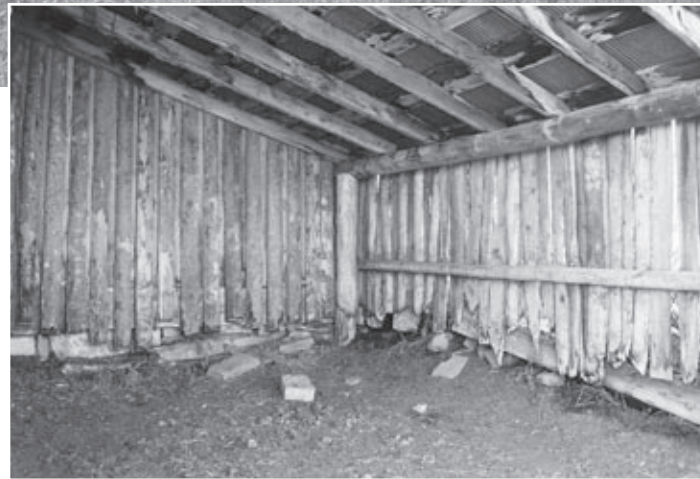
Top: A view showing the banking of the barn into the hillside. Bottom left: Inside the northeast corner of the lean-to, showing the stone foundation and the heavy timbers and planking of the walls.
