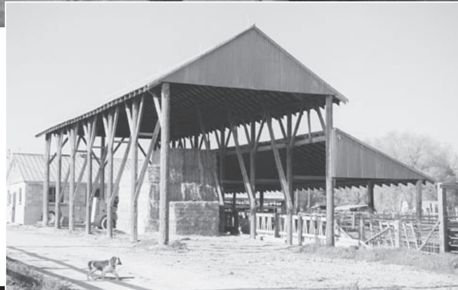
Top: The Liberty Lumber crew on a parade float. Left to right, they are DeVerl Passey, Vernon Parker, Fayon Pugmire, DeWain Passey, Don Hemmert, Stanley Morgan, and Hulme Matthews. Bottom: A hay shed in Newton, Utah, built by Liberty Lumber and Building.
