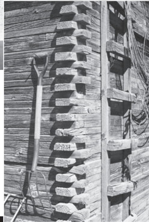
Top: Bucket milkers hang on the wall of the milking parlor. Bottom: A closeup of the corner of the granary showing the joints of the horizontal 2x4s.
