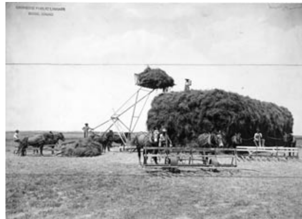
Upper left: A sheep barn completely sheathed in metal in Liberty. Lower left: A Jackson fork hangs in the rafters of an old barn. Upper right: Milking with a bucket milker. Photo courtesy Idaho State Historical Society, 1158-28. Lower: Building a haystack with an overshot hay stacker. Photo courtesy Idaho State Historical Society, 74.75.19.
